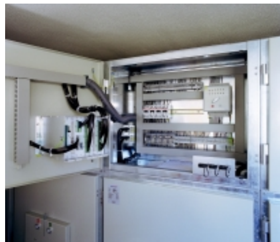
Figure 2: Reduced Wiring inside MV Cubicle
